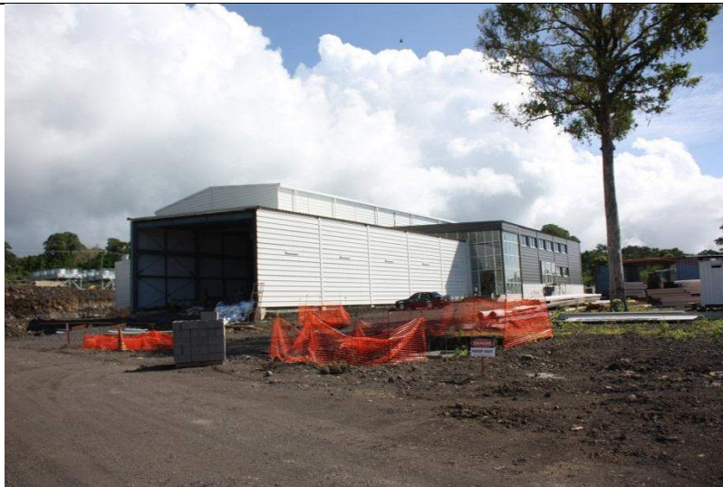
Above: Fiaga Power Station during construction works February 2012
